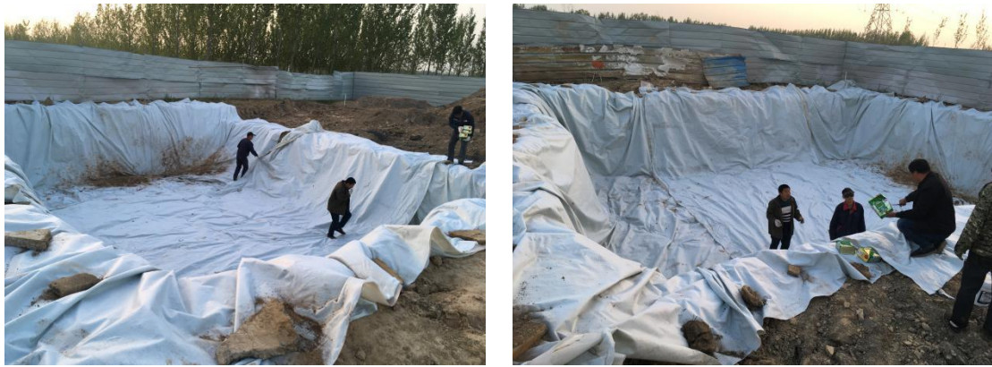
修复后土壤堆存区覆膜并用环保胶无缝粘接防渗
